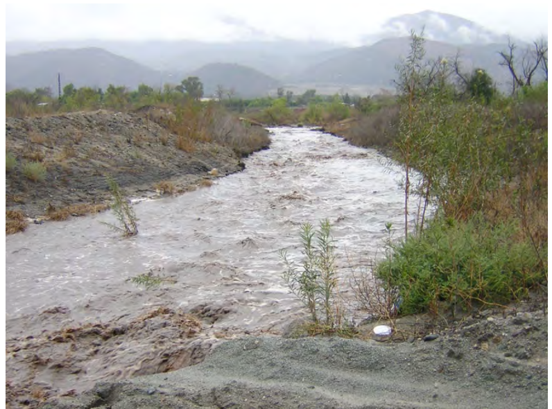
Flooding at Lilac Extension
