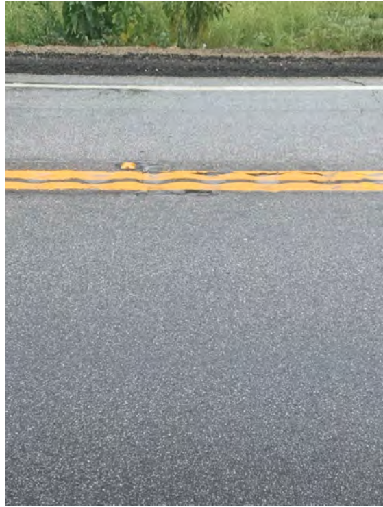
15 – Pala Mission @ Culvert and Camp Access
