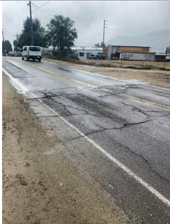
11 – Pala Temecula Road @ Trujillo Wash
