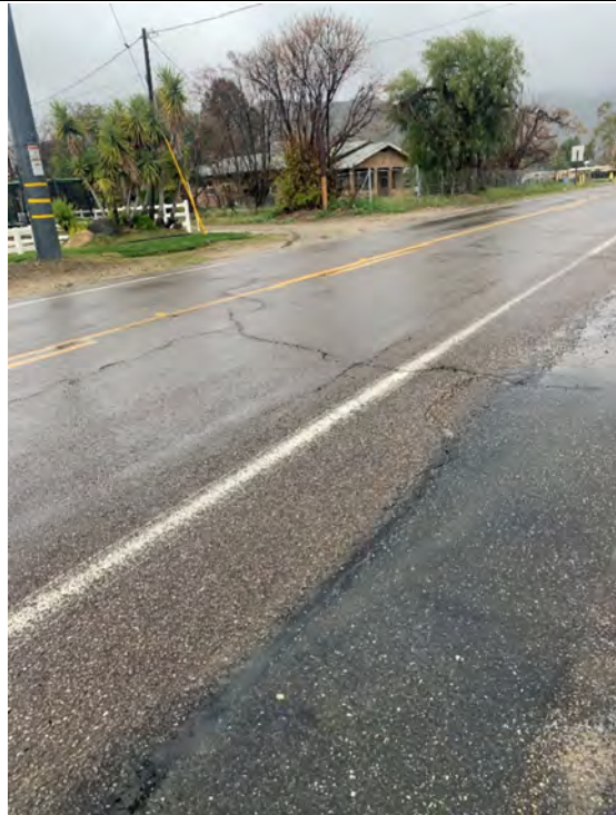
11 – Pala Temecula Road @ Trujillo Wash
