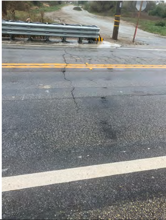
15 – Pala Mission @ Culvert and Camp Access
